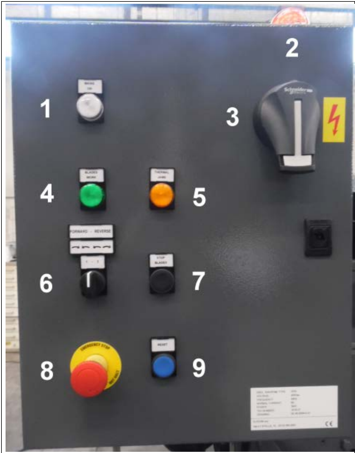
Figure 6-1 – Control panel lay-out (Current supply)
